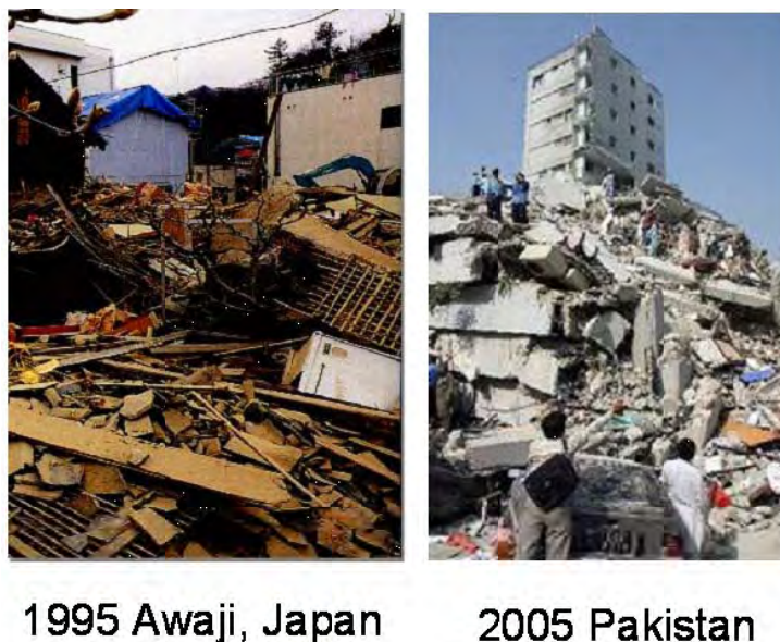
Fig. 1. Destruction examples of surface structures by large earthquakes
