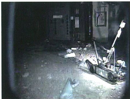
■ Figure 3: Examining inside reactor building with Packbots
