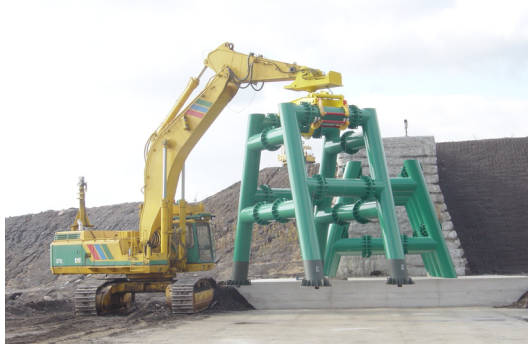
Fig. 2. Construction work status.
