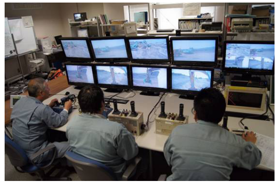
Fig. 12. Remote control room installed in remote Ministry of Land, Infrastructure, Transport and Tourism Office.
