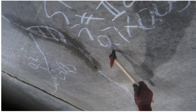
Fig. 1 Hammering test using an inspection hammer.
