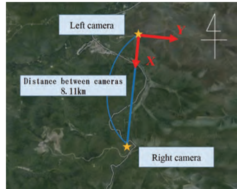
Fig. 8 The place where the cameras were installed
