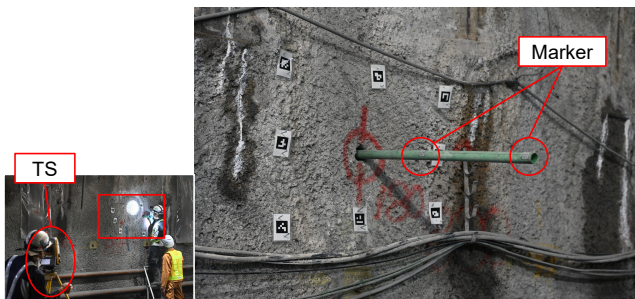
Fig. 10 Measurement using TS.
