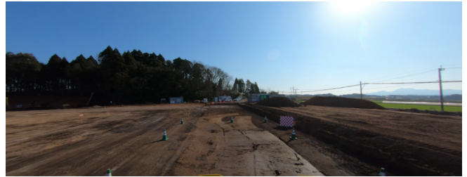
Fig. 1. A typical construction site scene in our setting
