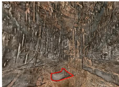
Fig. 2. Actual situation of the structure above the pedestal [2], to clearly show the location and state of the hole, we modified the figure by circling the hole at the bottom of the diagram with a red line.
