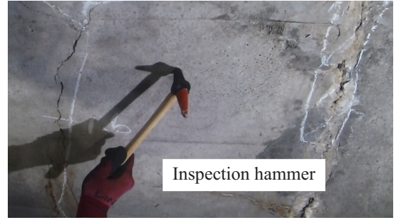
Fig.1 Hammering test and a inspection hammer
