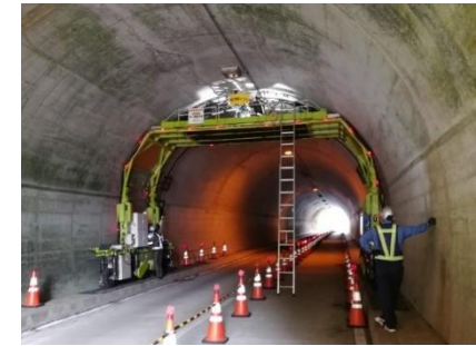
Robot inspection of tunnel
