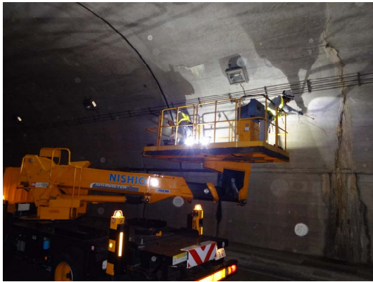
Fig. 1. Inspection by professional workers.
