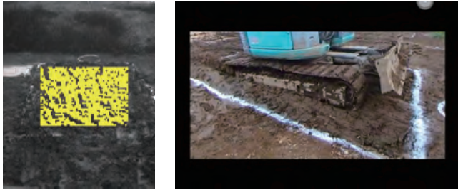
(a) Judgment result (b) Driving on soft ground by construction machine
